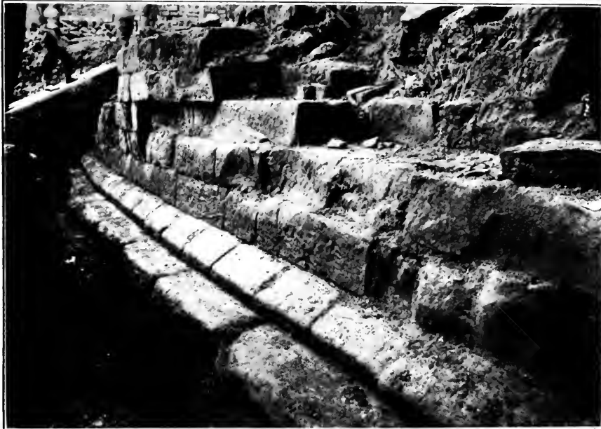
FIG. 4.—ROMAN WALL, LOOKING SOUTH. FOUNDATIONS BELOW FOOTINGS NOT EXPOSED.
